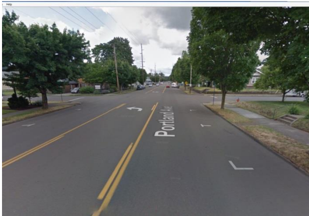
Portland Avenue, Facing South
