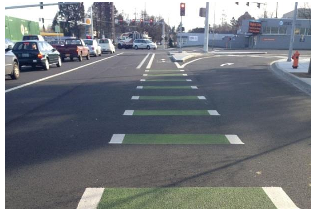
Pavement Markings Through Intersection
