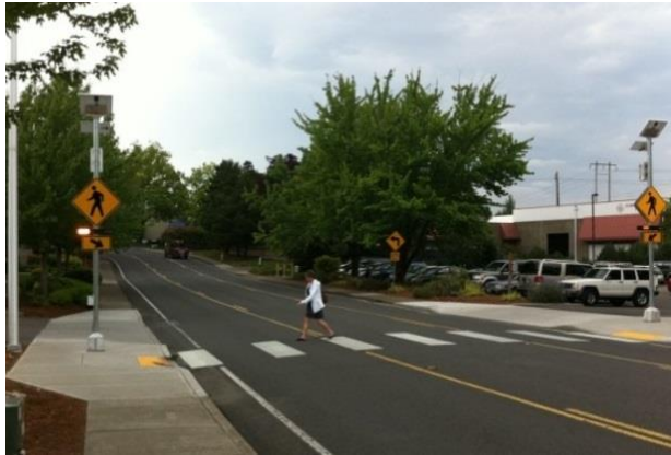
Enhanced Pedestrian Crossing with RRFBs
