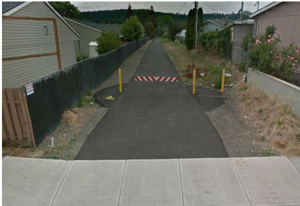
Existing Shared-use Path
