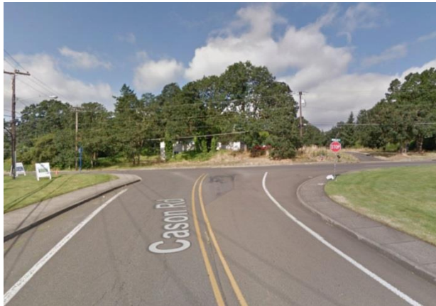
Cason Road, Facing West
