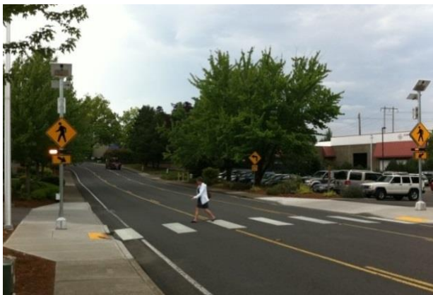
Enhanced Pedestrian Crossing with RRFBs
