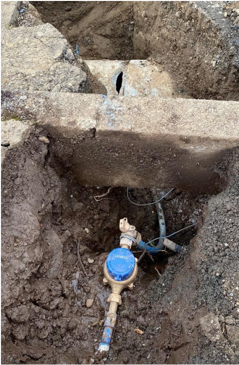
Water service repaired, Storm line repair addressed with a grout sealant that seals up holes as well as the separation that was evident at the joint.
