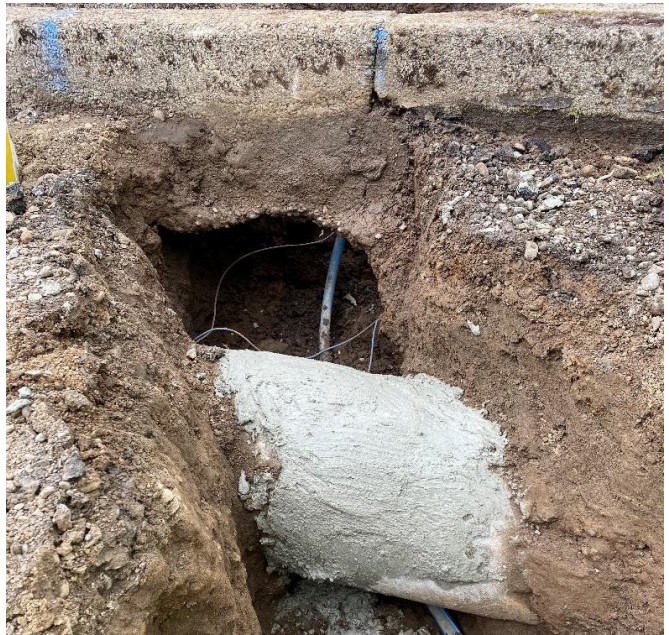
Water service repaired, Storm line repair addressed with a grout sealant that seals up holes as well as the separation that was evident at the joint.
