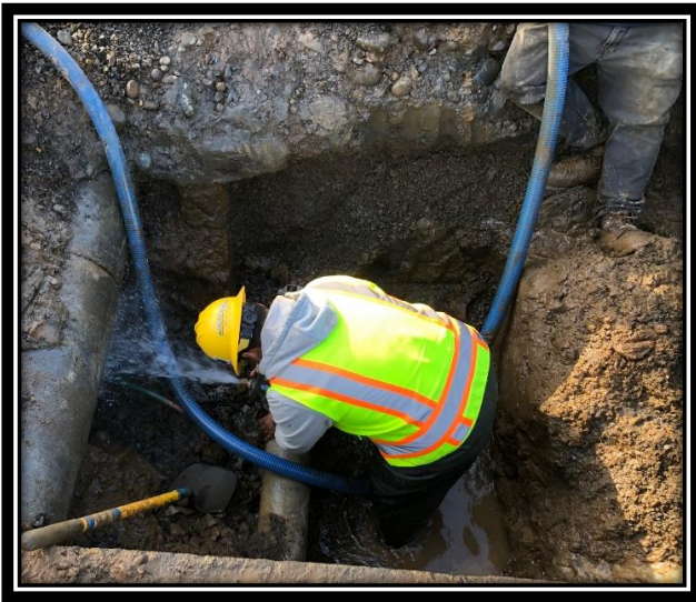
Crews work to repair a broken 6" transite water main and replaced a \frac{3}{4} " copper water service at 500 E. Kenmore Ave.
