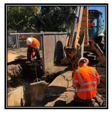
The crew uncovered and relocated the Cornell bike path 8" pressure reducing valve vault lid. The access hole was originally in a customer's back yard. Repositioning the vault lid so that the PRV is accessible in the bike path which is within the City ROW instead of on private property.
