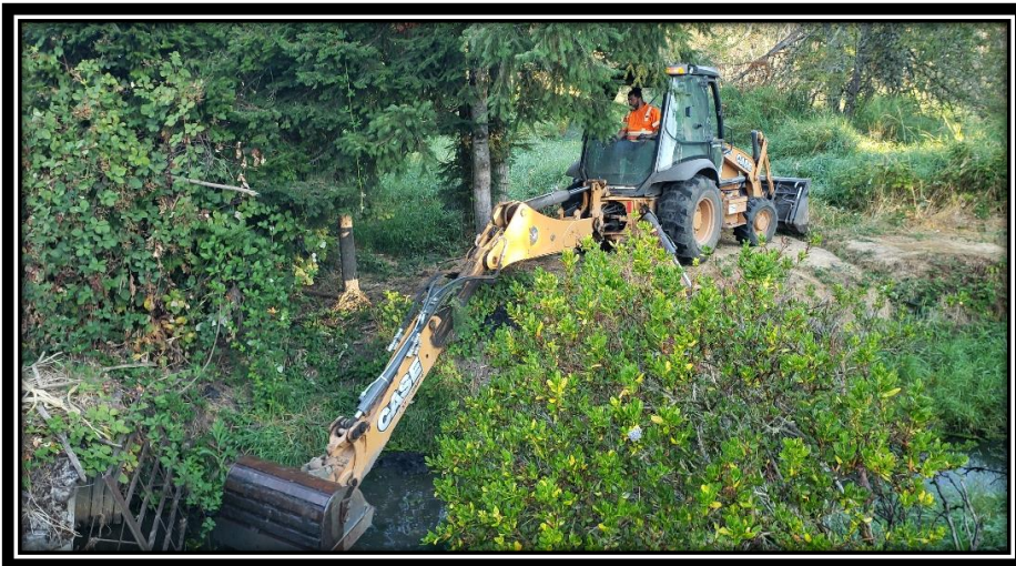
(Cleaning out debris at headwall of the Risley Ditch).
