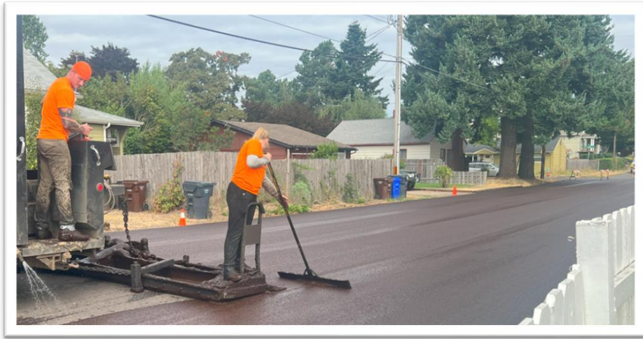
The Annual Slurry Seal Project, crews from Blackline, Inc. work to apply the slurry seal emulsion on Barton Ave.
