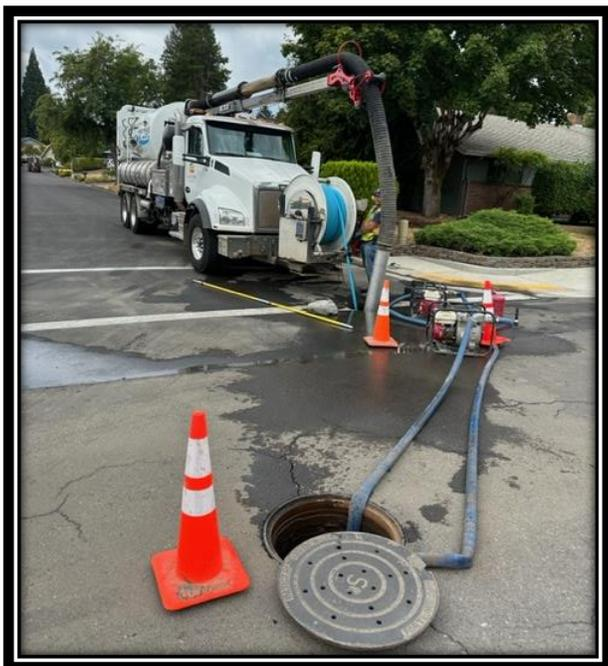
The Barclay Stormline project is coming up on the end of its maintenance bond period requiring an inspection of the projects main components. Crews jetted, cleaned and CCTV'd the new stormline on Barclay from Portland Ave to Watts Ave.
