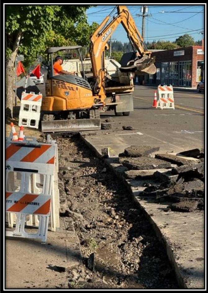
The Water Dept. had what appeared to be a small water leak that turned into a substantial job that included two taps that serve three businesses and one residence. The repair took crews several days to complete with challenges due to the location and other ongoing construction projects in the area.
