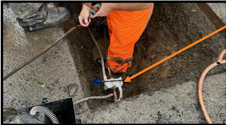
Frozen water line, which allows crews to replace the valve.
