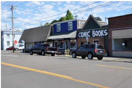
On-street parking maintained on Portland Avenue and reconfigured in the Downtown Core segments due to a street redesign.
