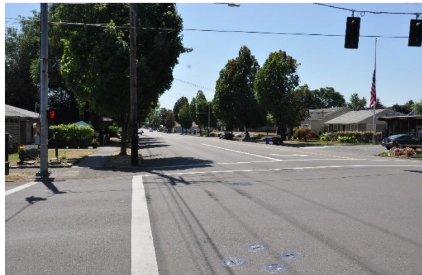
6: Portland Avenue overall, with wide curb-to-curb and lane widths, could benefit from a road diet that slows speeds, provides ped/bike facilities, and improves landscaping and stormwater management while maintaining room for cars, parking, and transit.
