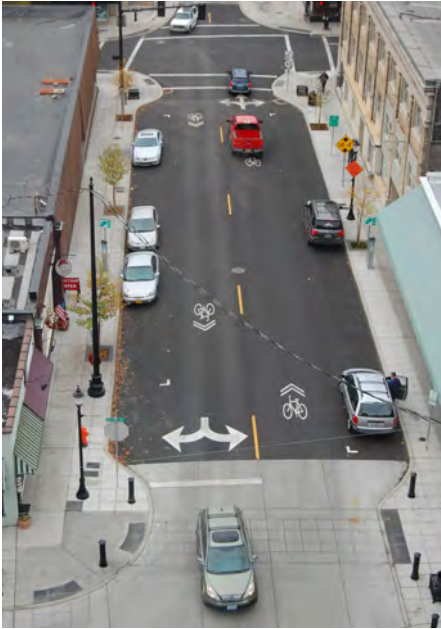
A shared street environment with wide sidewalks, parking, and intersection design treatments. (Oregon City, OR)
