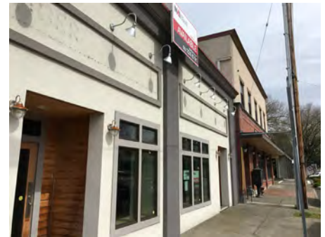
Storefront improvement adds new life to tired commercial buildings. (Milwaukie, OR)
