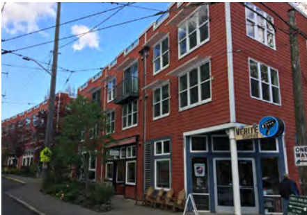
Mixed-use housing over retail development can occupy fairly small 1/4 and 1/2 block lots. Code revisions in Gladstone will allow additional first-floor heights. (Madrona - Seattle, WA)
