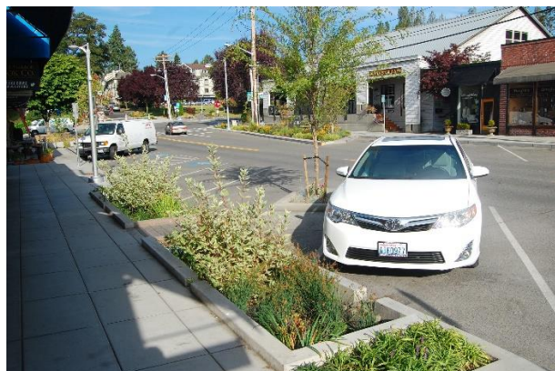
Road Diet and Character: This example 70-foot right-of-way street was slimmed down with wide sidewalks, stormwater facilities, angle parking, and other humanizing elements. (Bainbridge Island, WA)
