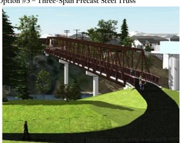
A three-span bridge was considered because it is one of the most common types of bridge structures in Oregon. The total project cost is estimated to be \$5.5 million in today's dollars, which is the very middle of the alternatives. The bridge would be harder to permit because of the columns in the river.
