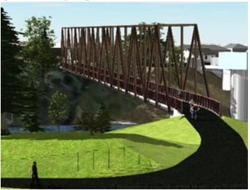
A steel truss bridge was considered because it is similar to the previous bridge. The total project cost is estimated to be \$6.6 million in today's dollars, which is second highest amongst the alternatives. The bridge would be the easiest to permit because no columns would be in the river.
