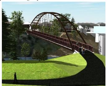
A single-span steel arch bridge was considered because of its aesthetic qualities. The total project cost is estimated to be \$10.9 million in today's dollars, which is the highest amongst the alternatives. The bridge would be the easiest to permit because no columns would be in the river.
