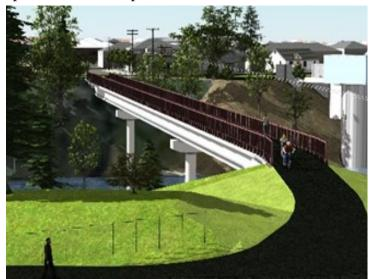
A precast, pre-stressed concrete bridge was considered because it is a common type of bridge structure in Oregon. The total project cost is estimated to be \$4.9 million in today's dollars, which is the lowest amongst the alternatives. The bridge would be harder to permit because of the columns in the river.
