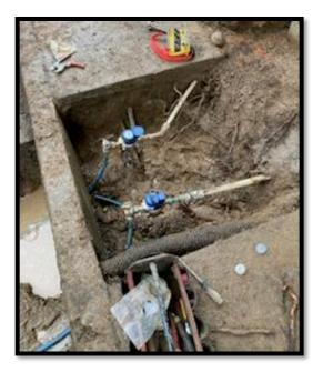
Crews discovered leaking water service lines on Parkway after noticing water in the roadway. Crews replaced both of the independent service lines and placed a repair band on the service line that is off of the city water main. Crews utilized the line-freezing machine to perform repairs.
