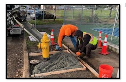
Per City Standards, crews poured a concrete pad around the recently installed fire hydrant on E. Exeter near the courts at Max Patterson Park. The hydrant replacement portion of this project was completed in October, the hydrant was identified for replacement due to the hydrant containing large amount of lead as well as the hydrant not having isolation gate valves. With the installation of the hydrant pad, this project is now completed.
