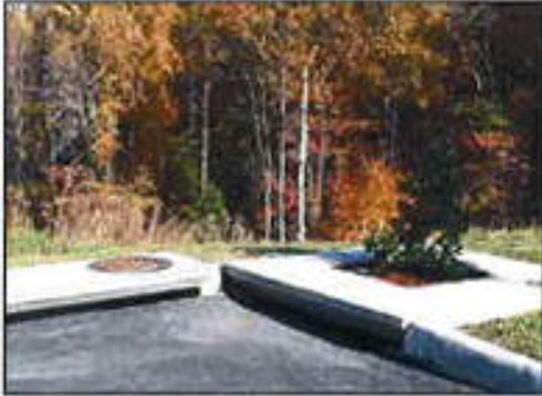
1. Inspection of Filterra and surrounding area
