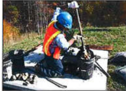
2. Removal of tree grate and erosion control stones
