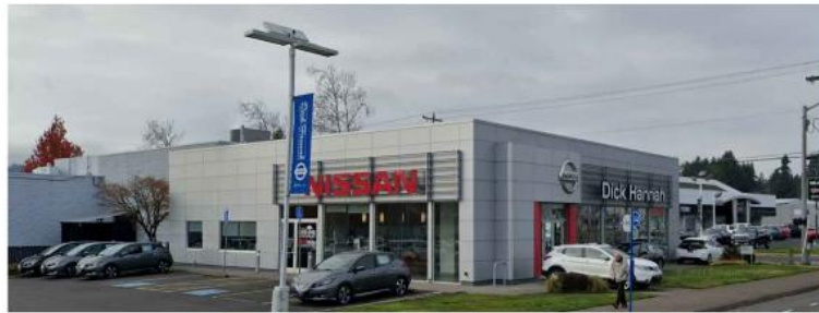
EXISTING SOUTH FACADE 4.
