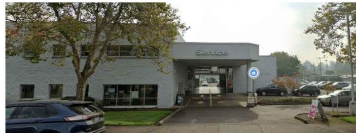
EXISTING NORTH FACADE 2.
