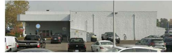
EXISTING WEST FACADE 3.
