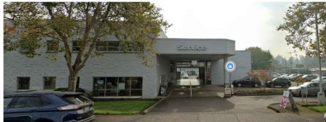
EXISTING NORTH FACADE 2.
