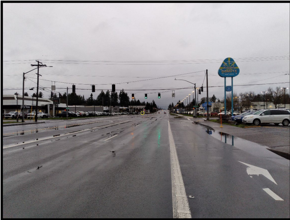
Figure 5: Viewing North to the Northwest Access (Access #1)
