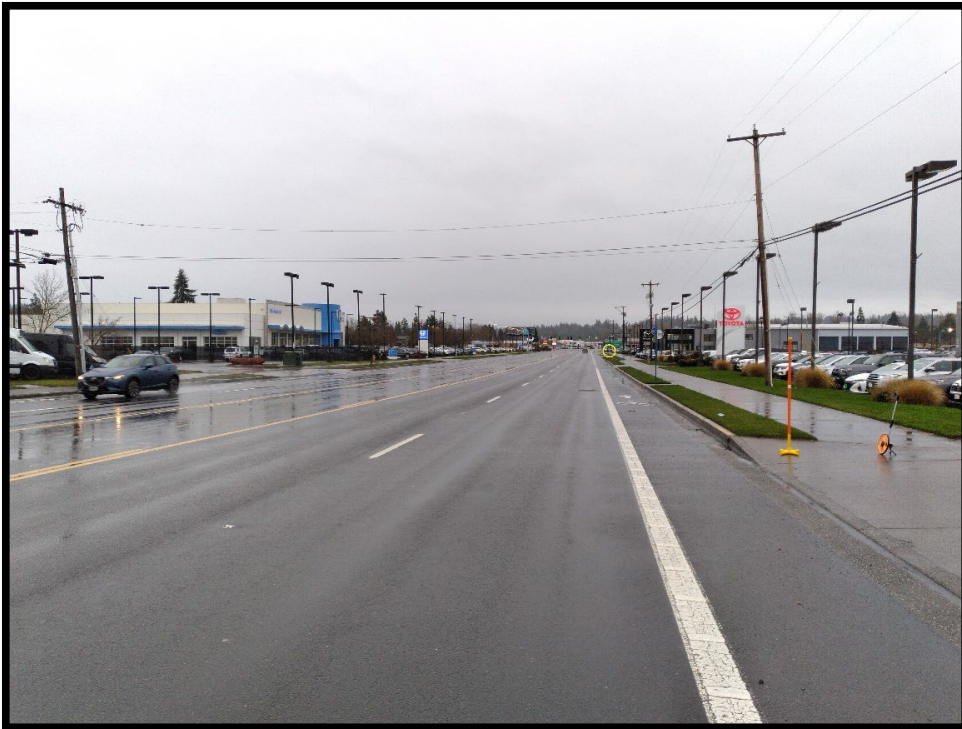
Figure 7: Viewing South to the Southeast Access (Access #2)
