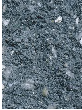
CMU-1 Concrete Masonry Unit, Exterior Perimeter of Building
