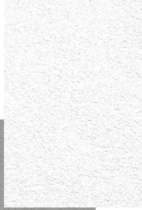
EIFS-2 Exterior Insulating Finishing System, Exterior Rear Facade
