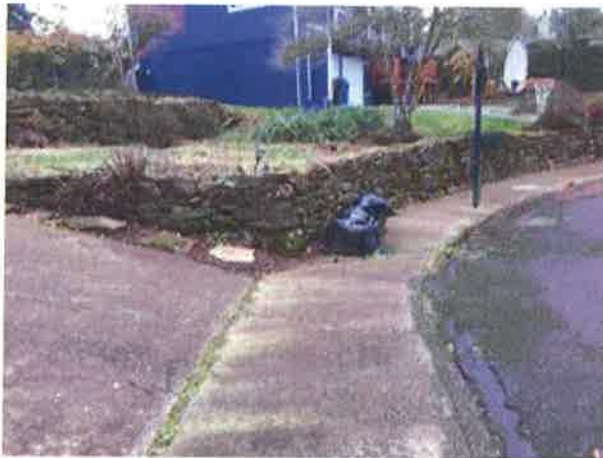
Collins Crest – Prohibited Garbage Storage
