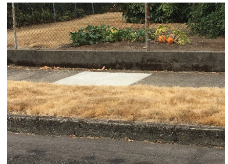
Exeter Sidewalk After
