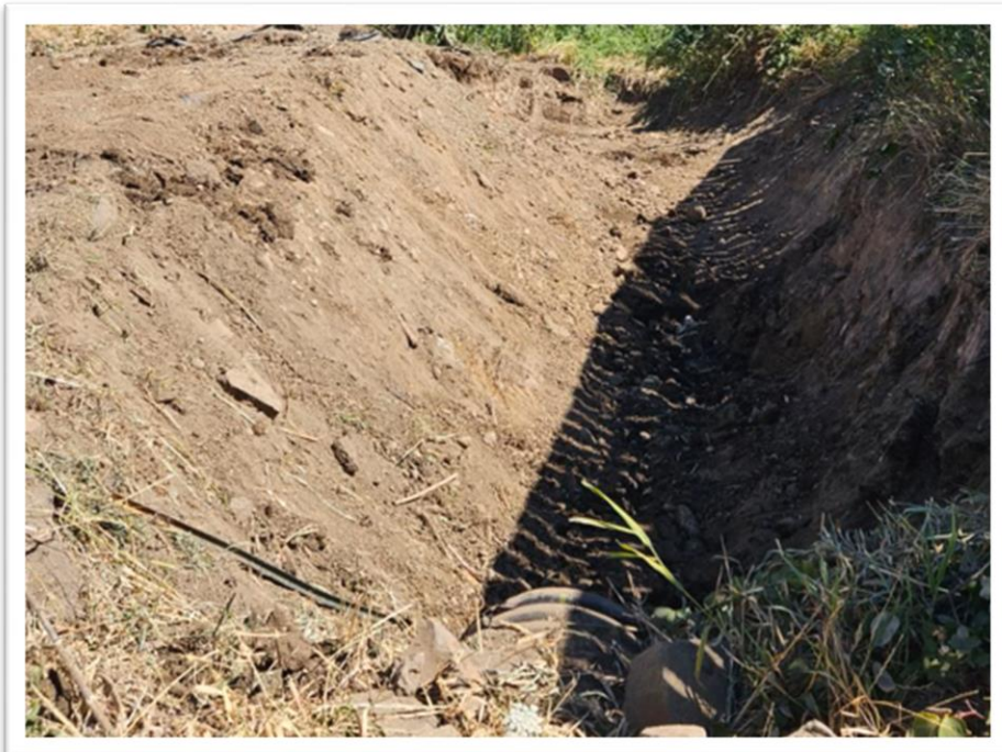
Dugout the ditch coming from Glen Echo which floods the road, below
