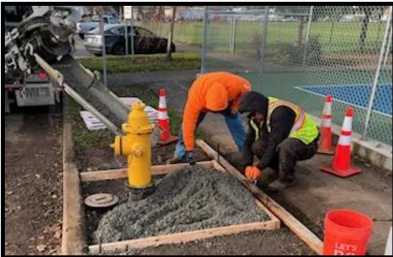
Per City Standards, crews poured a concrete pad around the recently installed fire hydrant on E. Exeter near the courts at Max Patterson Park. The hydrant replacement portion of this project was completed in October, the hydrant was identified for replacement due to the hydrant containing large amount of lead as well as the hydrant not having isolation gate valves. With the installation of the hydrant pad, this project is now completed.
