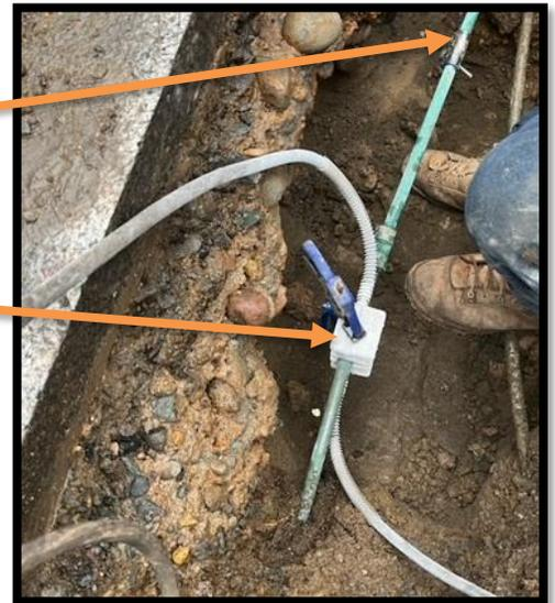
The freezing machine was placed on the main service line, which is installed off the water main. This line in this case then splits into two independently metered service lines for the residents
