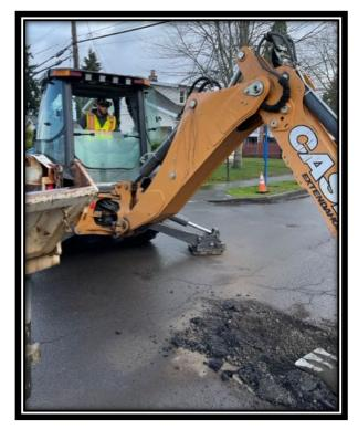
Crews responded to reports of a sink hole in the area of Arlington @ Beatrice, a location that we have responded to before for the same reason. Crews removed the roadway and utilized the vactor truck to hydro-excavate the area to ensure that there were no additional voids causing the sinking. Crews added compacted rock to the hole and repaved the area within the roadway. Crews were able to determine that there was no underlying reason for the sink hole, such as a water line break
