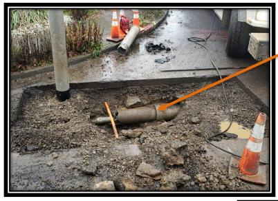
Pictured to the left is the stormline with the smaller pipe connected to the larger pipe which causes a reduction in flow.
