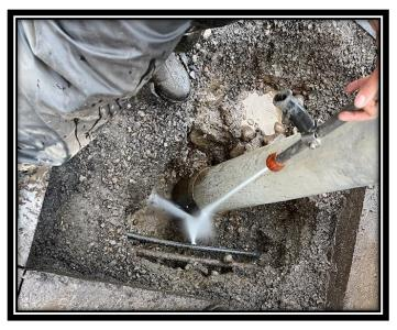
Crews responded to reports of pooling water on the roadway near 260 Harvard Ave. Utilizing the Vactor truck crews hydroexcavated to locate the leak and placed a repair clamp on the water line.
