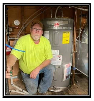
Crewmember Rex McIntire worked to replace the hot water heater at the Fire Department, the old one began to leak in the attic space.
