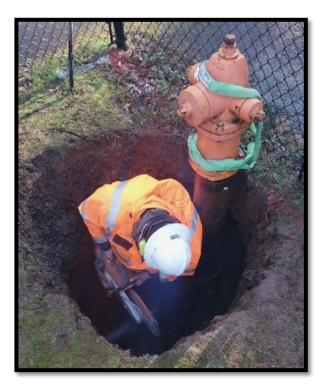
Crews relocated a fire hydrant that is located at the Kirkwood Reservoir. This hydrant was identified as needing to be relocated due to the access being limited, being located to close to the existing fence limited the ability to wrench the hydrant open without interference. Relocating the hydrant resolves this interference and will make the hydrant fully accessible in the case of an emergency.
