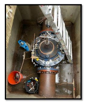
Installed control valves to an existing altitude valve at the Webster pump station. This valve installation will allow crews to better control the rate of which water fills the reservoirs in case of an emergency. (pictured left)
