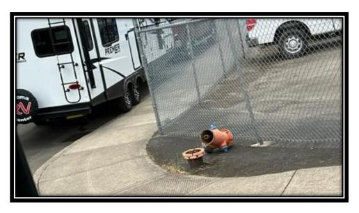
The Water crew repaired a water leak at 335 Patricia Drive, using the vactor truck to hydro-excavate the site, crews were able to make a timely repair on this dual service line.
