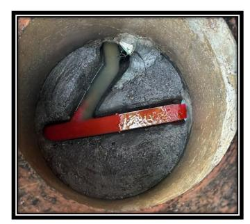
Sewer crews responded to a sewer backup at Gladstone Toyota, to assist in the investigation crews used red dye to verify that the lines were running clear on the City side.
