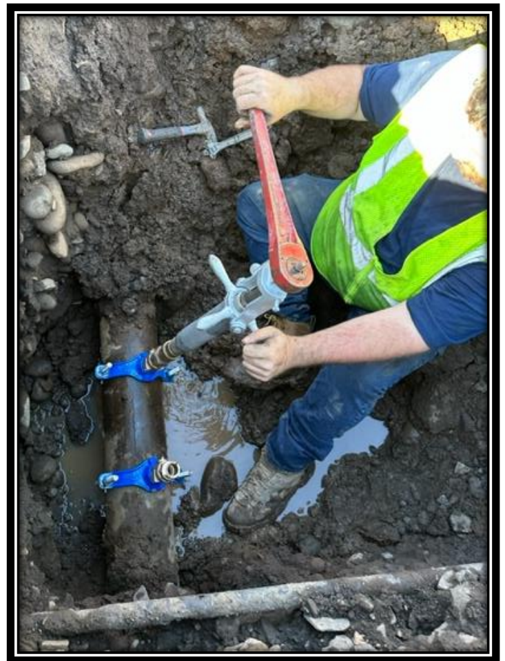
Crewmember Eric Fanning using the tapping machine to re-tap the water main for the new service lines on Portland Ave. (Pictured right)
