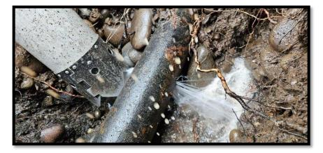
Crews have stayed busy with plenty of water repairs and service replacements recently. The service line at 510 E. Arlington was replaced due to the significant break in the line, which could not be repaired adequately.
