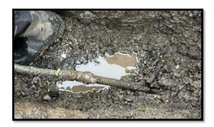
Crews also repaired a leak on a main key valve on Hanson Ct. Replacing the lever valve had it back in service quickly.
