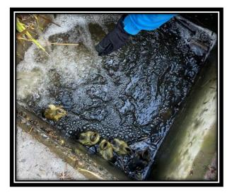
Crews repaired a 12" storm line on Portland Ave. that was causing sinkhole due to improper installation. Crews utilized the Vactor truck to excavate the area around the pipe to locate the damaged section. Once identified crews were able to remove the damaged piece of pipe and section in a replacement piece, properly backfilled and compacted the area and wrapped up the repair.
