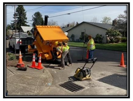
The Streets Department recently purchased a Hot Box, this piece of equipment will allow crews to have hot mix ready and on demand for patching utility cuts and to make other patching repairs when needed. Once the weather improves a bit we will have this new equipment out regularly doing more patching projects. This is a great investment for the City and the streets department can't wait for the drier days of late spring to be here so they can get it out more frequently!
