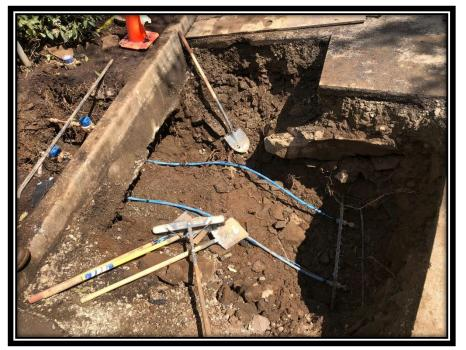
Crews replaced two leaking  $\frac{3}{4}$ " black poly material water services on Patricia Dr. This has been an ongoing leak which we were finally able to locate after an ongoing investigation. Water leaks are not always easy to find, water finds the path of least resistance and it can take a while to track it back to the source. Many residents on Patricia will be happy that this has been resolved.
