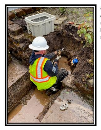
Crew member Jeff Shepherd working to move the water meter to the edge of ROW, working behind the customers retaining wall in order to minimize disturbances as much as possible. The finished product looked great and we no longer have a water meter in the middle of the roadway!
