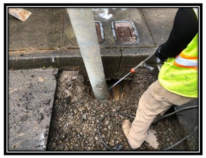
The Water crew works to repair a leaking 3/4' service on Monticello Dr. Using the Vactor truck to assist in excavating the area using pressurized water and the strong suction from the Vactor truck crews can minimize disruption to the area while accessing the lines in which need to be repaired.
