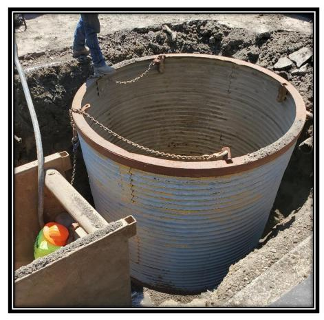
Crew members from Jim Smith Excavation have shoring in place, preparing for the installation of a new manhole on Barclay Ave.
