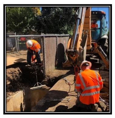
The crew uncovered and relocated the Cornell bike path 8" pressure reducing valve vault lid. The access hole was originally in a customer's back yard. Repositioning the vault lid so that the PRV is accessible in the bike path which is within the City ROW instead of on private property.
