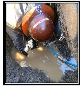
Crews responded to a water service leak on Hardaway Ct. This 1" PVC black poly material line has experienced multiple leaks/repairs in the past. Faulty pipe material appears to be the cause of repeated failures and leaks. We repaired the current leak and put the entire service line on the maintenance schedule.
