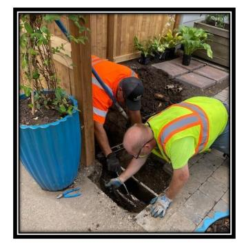
Crews worked to repair an irrigation line at the Senior Center that was damaged within the new garden area. The line was near a newly installed fence post and appears to have been damaged by the contractor.
