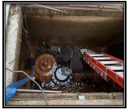
GC Systems performed routine maintenance on the 8" and 2.5" pressure reducing valves on Valley View Dr. These valves serve as an intertie with Oak Lodge and open up to allow water into the high zone when they sense a drop in pressure as result of fire flows or pump failure etc.
