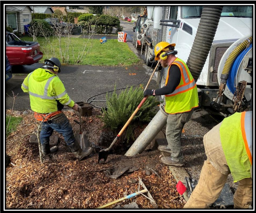
Crews replaced a \frac{3}{4} " water service on E. Exeter St. which contained a broken curb stop.
