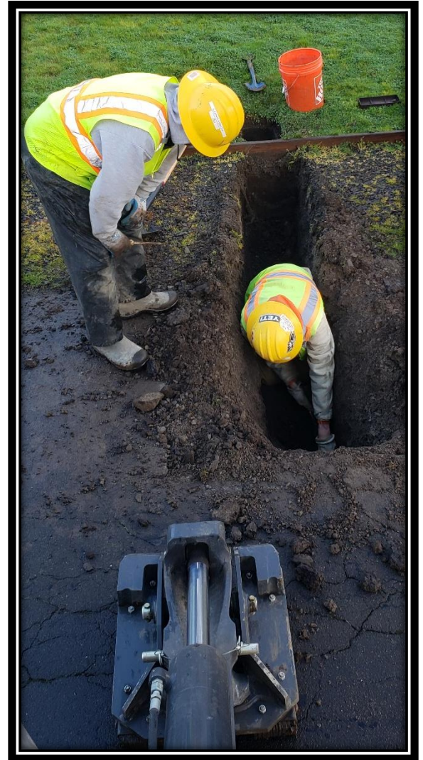
Crews replaced a \frac{3}{4} " water service on E. Exeter St. which contained a broken curb stop.
