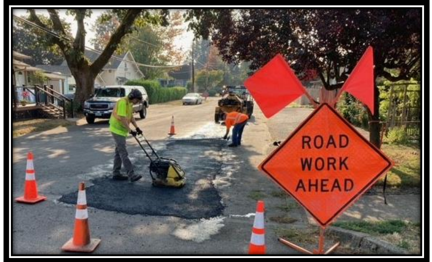
Skin patching (paving) continued, crews laid down 8.25 tons of asphalt on Beatrice Ave.
